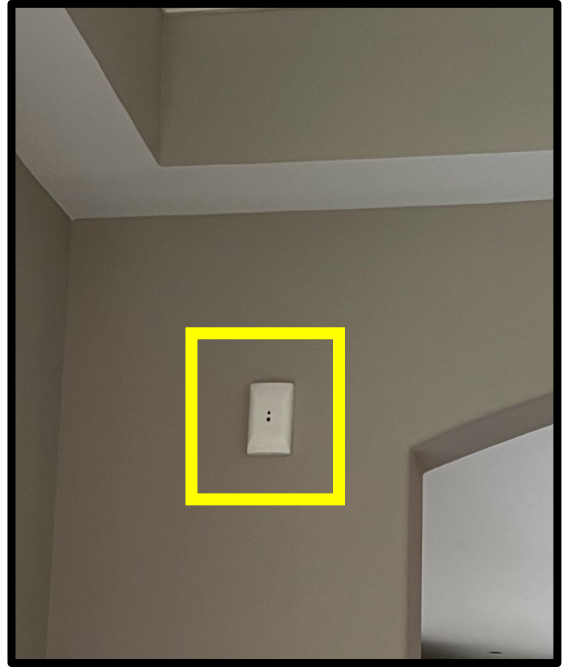
Example of wall mounted acoustic glass-break sensor.
